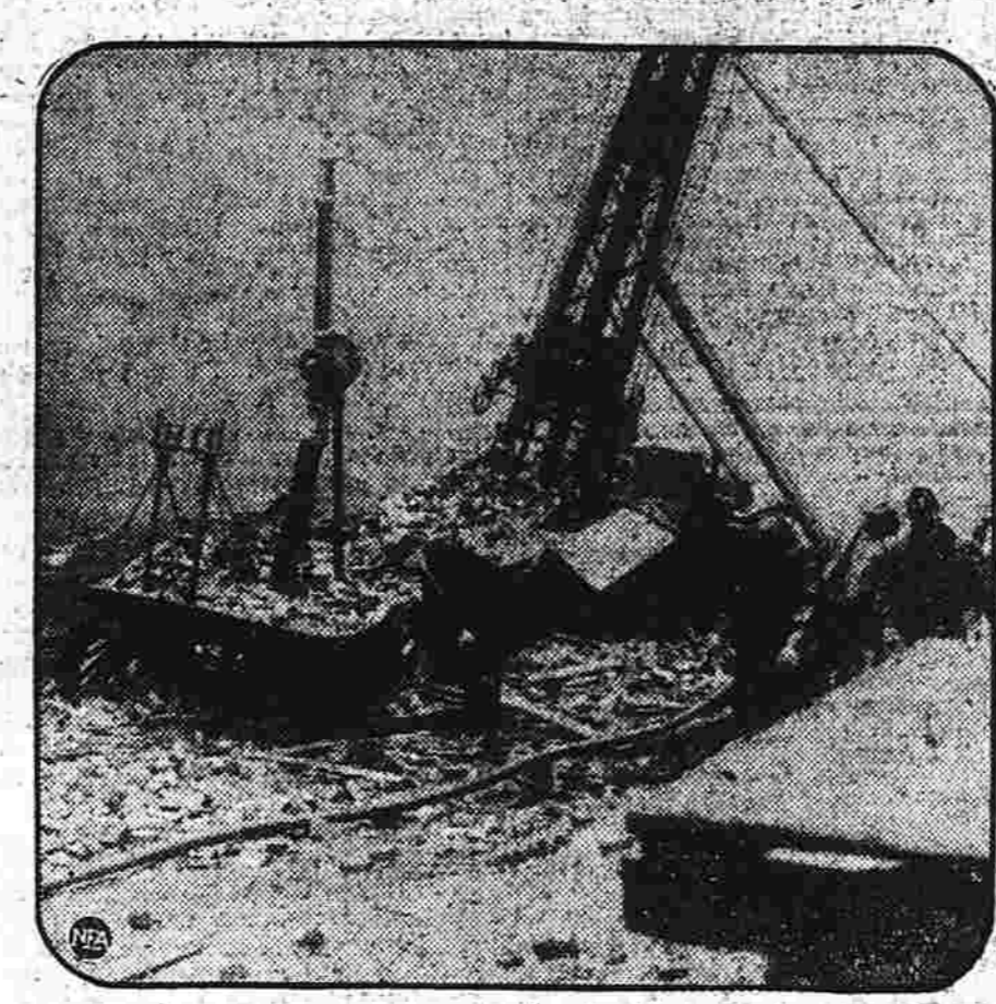
This was a $20,000 fire-fighting water tower—before a falling wall hit it during a spectacular auto warehouse blaze in New York. The water tower crew escaped with injuries to only one. Two million dollars in property, including 800 cars, was destroyed before the fire was subdued.
